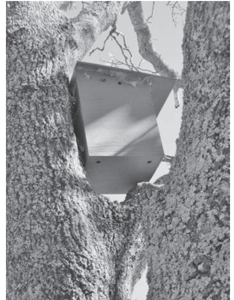
At the curbside tree next to the retaining wall and driveway of 57 Club View.
