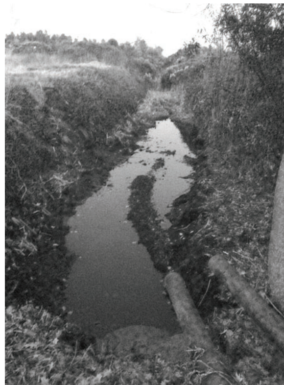
V-ditch behind Club View Drive
