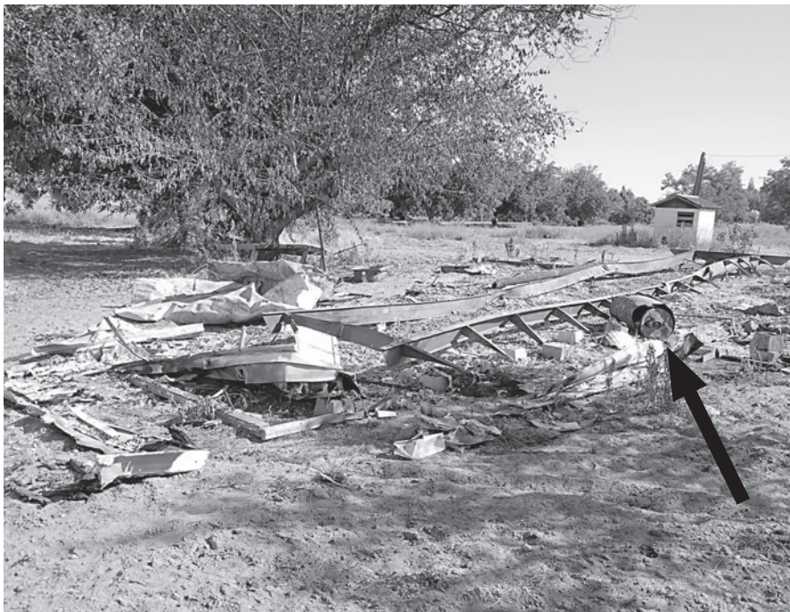
The remains of a mobile home fire from a faulty water heater.
