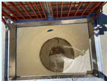
Pump Station Interior with New Polyurethane Coating
