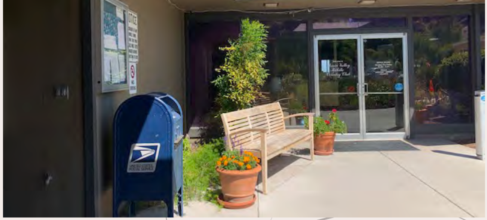
Clubhouse Entrance - Part Sun
